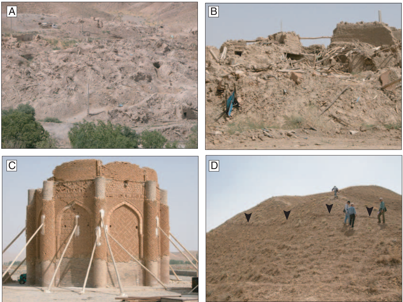
Figure 4. (a) Photograph looking roughly north from 35^{\circ}47'41.5''\text{N} , 49^{\circ}07'22.9''\text{E} at earthquake damage at Abdarreh. (b) Close-up of earthquake damage to single-storied adobe housing at Abdarreh. (c) Kharaqan Seljuk domed mausoleum near Hesar ( 35^{\circ}50'27''\text{N} , 48^{\circ}57'40''\text{E} , see Fig. 3 for location), damaged during the 2002 Changureh earthquake. (d) Thrust ruptures observed near Abdarreh village at 35^{\circ}47'41.5''\text{N} , 49^{\circ}07'22.9''\text{E} .
